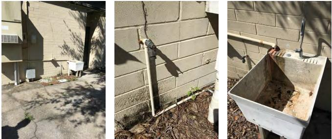
**Figures 25, 26, and 27** - These photos show the exterior utility sink installation and condition. The piping for both domestic water and sanitary waste and vent is pvc and is exposed to the elements and to damage. The sink is in poor condition and is used as a receptacle for condensate from the adjacent wall mounted A/C unit. There is a hose bib located near the sink which is also served by exposed pvc piping. The sink is vented by an air admittance valve located next to the sink.
