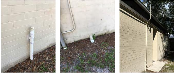
**Figures 31, 32, and 33** - These photos show typical external waste and vent piping that was installed to serve fixtures added in renovations subsequent to the building's original construction. There are several locations where exterior pvc waste piping was added to serve miscellaneous sinks inside the building with venting being done with air admittance valves. The pvc piping is exposed to weather and the elements and is subject to degradation and damage.
