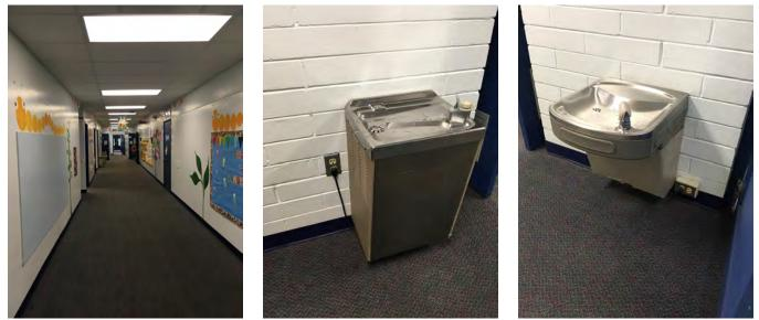
Figures 16, 17, and 18 - These photos show the locations of the two interior electric water coolers and their condition. The casing on both units show signs of rusting and deterioration.
