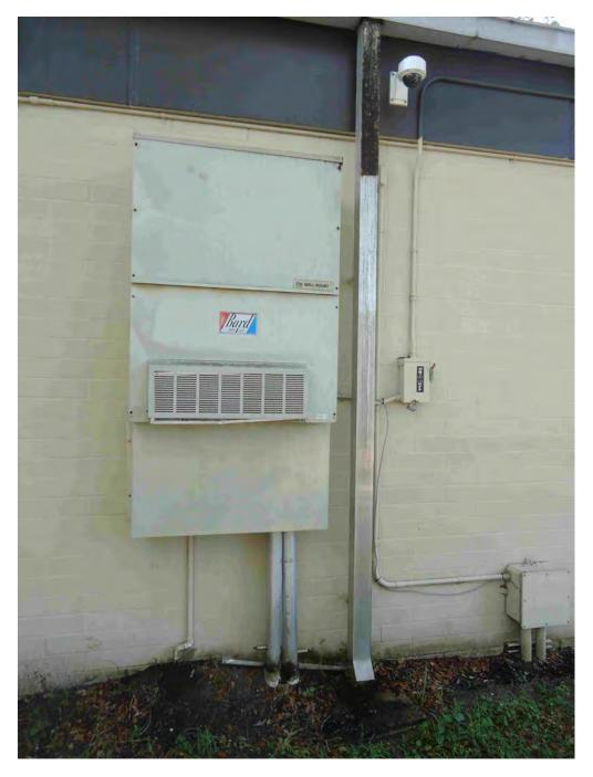
Exterior wall mounted Bard A/C unit showing damaged outdoor air intake grille and condensate drain.
