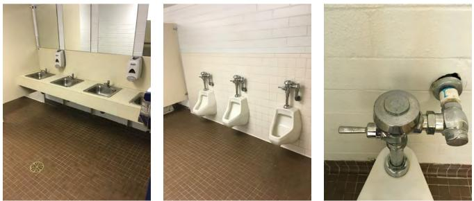
**Figures 1, 2, and 3** - Condition of the fixtures in the Boy's Group Restroom. The fixtures are a mixture of white vitreous china and stainless steel. There is not a designated ADA lavatory or any protective piping covers. The lavatory faucets in this restroom are all of the metering type. There are grab rails at one of the water closets but there is not sufficient space to provide for wheel chair access or turnaround space.
