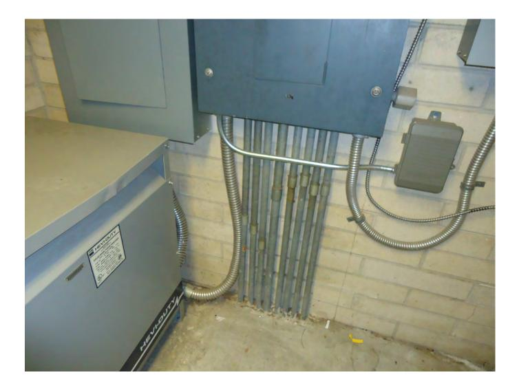
According to the best information available to the industry, electrical panelboards expected life is approximately 30 years. Therefore, the existing electrical gear is currently approaching 50% more than would typically be expected.
