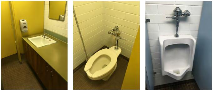
**Figures 13, 14, and 15** - These photos show the typical condition of the staff restrooms. Again, none of the fixtures in either the Women's or the Men's staff restrooms appear to be compliant with current ADA requirements, nor does there appear to be space to address ADA clearance issues.
