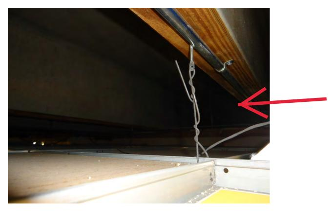
Photo shows limited space between lay in ceiling and structure.
