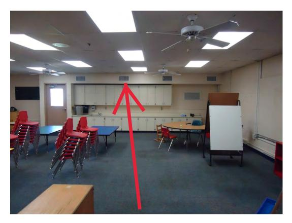
Interior view of typical classroom showing four supply registers within a soffit below the ceiling and the wall mounted return grille. Bard unit is directly behind the return grille.
