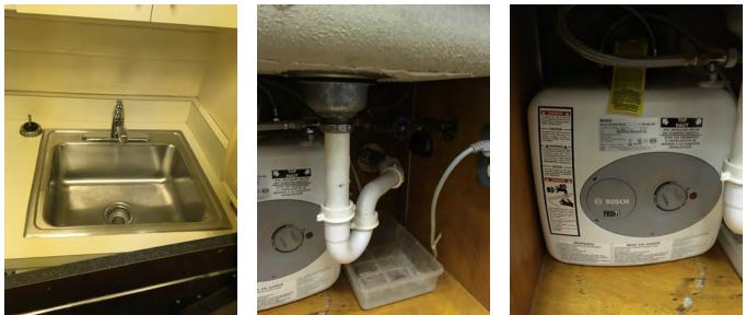
**Figures 22, 23, and 24** - These photos show the sink and water heater installed in Room 005B. The sink is a stainless steel countertop model with a single handle faucet. The water heater is a Bosch Model ES 2.5-1M WIR S3100. The water heater is a 2.7 gallon unit with a single 1,440 watt heating element. Both the water heater and sink are in good condition.
