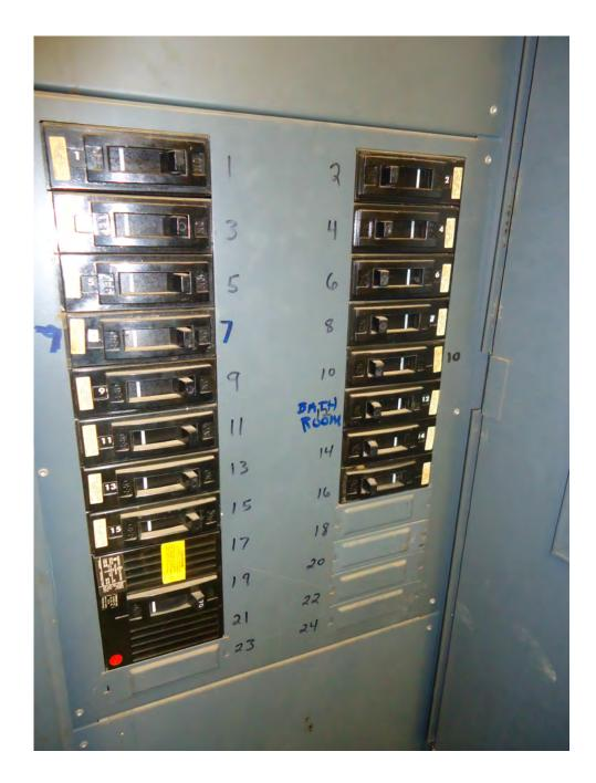
The existing electrical gear is currently installed in a custodial closet with limited space. The existing configuration of the electrical gear is not code compliant with regards to working clearances and working space. The lack of working clearances and working space has a direct bearing on the potential safety of facilities personnel when operating and maintaining the existing electrical gear.
