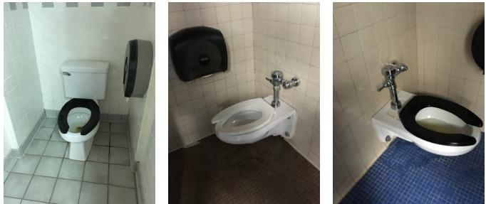
**Figures 7, 8, and 9** - These photos show the typical condition of the primary classroom unisex restroom water closets. There are no grab rails or wheelchair access. Figure 8 shows the flush handle to the far side of the water closet away from the access. There is a mixture of flush valves, flush tanks, wall mount water closets, and floor mount water closets. Figure 9 shows potential signs of leakage.
