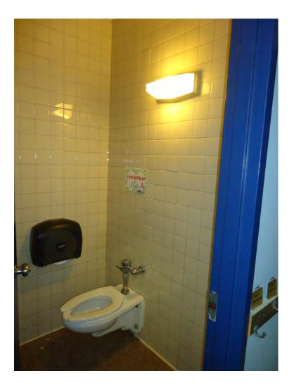
Most of the existing spaces that would typically require emergency egress lighting fixtures do not currently contain a fixture with battery backup (no emergency generator is existing on the campus). Overall, the existing emergency egress lighting appears to be deficient. The existing exit signage appears to be code compliant and not deficient.
